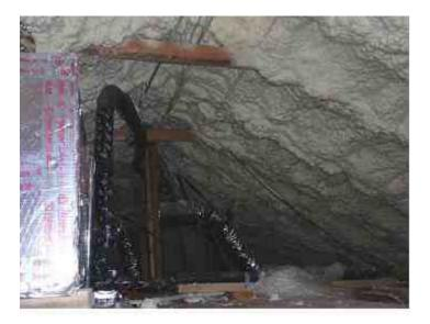
Have you ever encountered an attic which has sprayed foam applied to the underside of the decking? Then you notice that the foam extends into the cavity between the rafters at the top plate effectively sealing the attic. The bare drywall showing between the joists really looks weird and out of place doesn't it?
